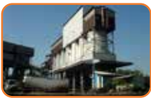
Land Cement Silo Cigading Serang, Banten Cigading Cement Silo Serang, Banten
